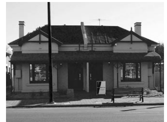
Unley Electorate Office
